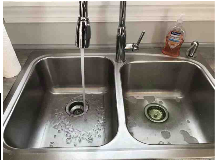
Utilities operational, no garbage disposal
